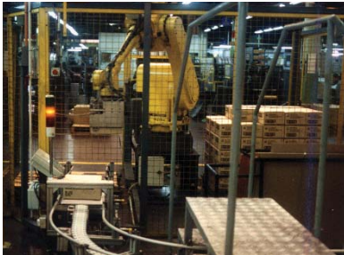
Conveyor System & Robotic Palletizing
