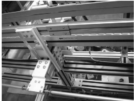
Automated side guide installed at straight section
