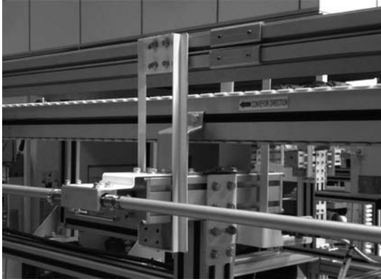
Automated side guide installed at straight section
