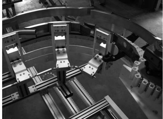
Automated side guide installed at bend section
